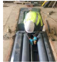
Installation to a prepared site
